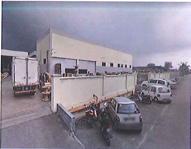
Rembia Industrial Park that is located at 3km west from the Project site
