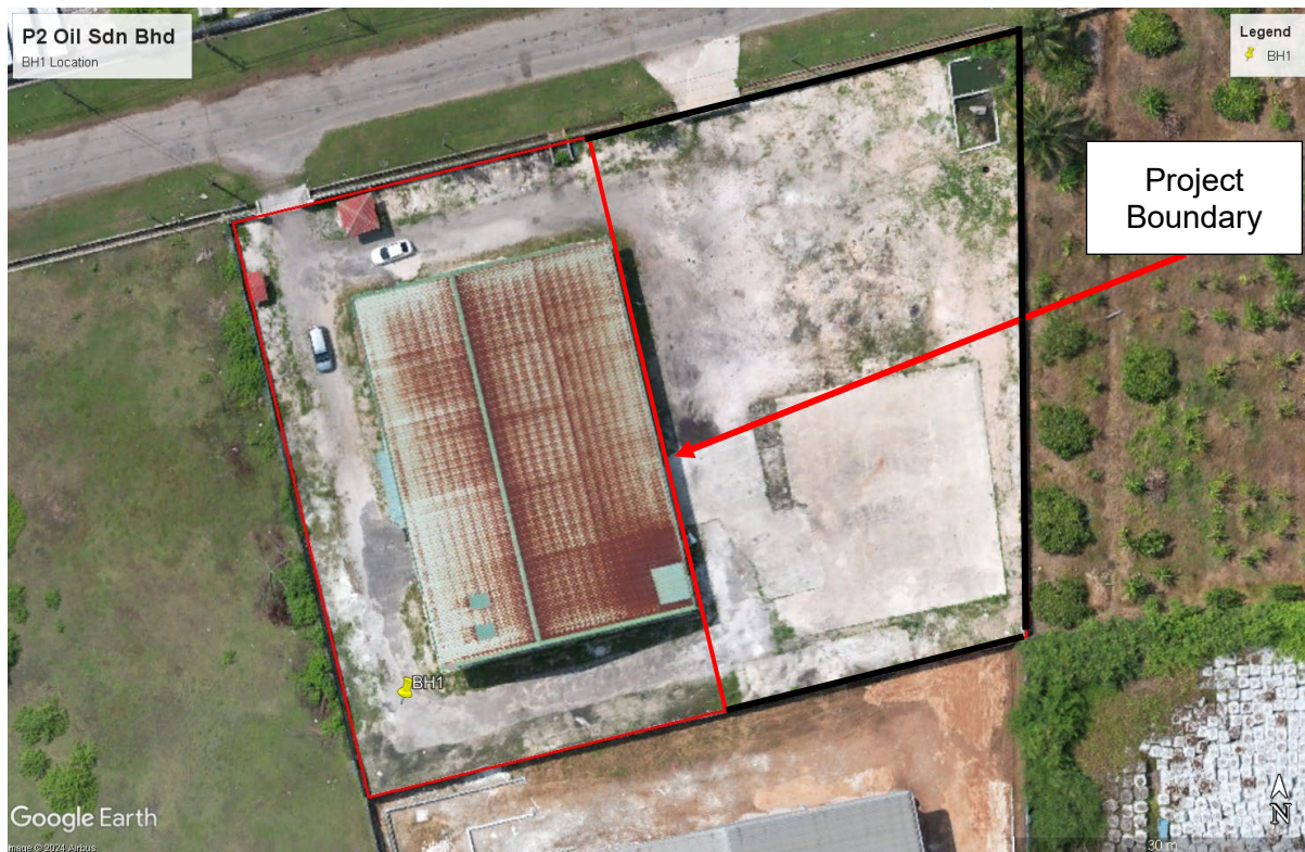
Figure 6.7: Monitoring Station for Groundwater Quality
